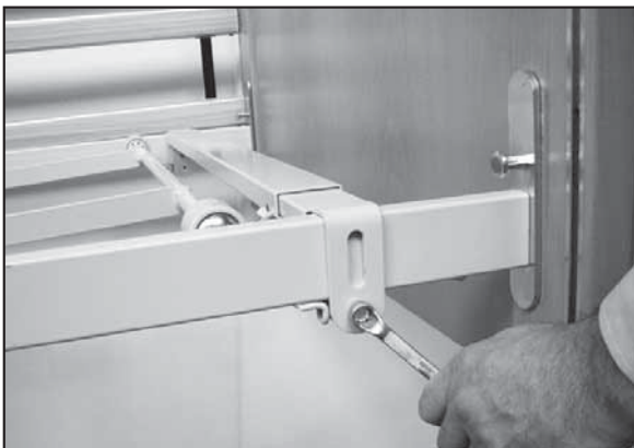
The screws are tightened
